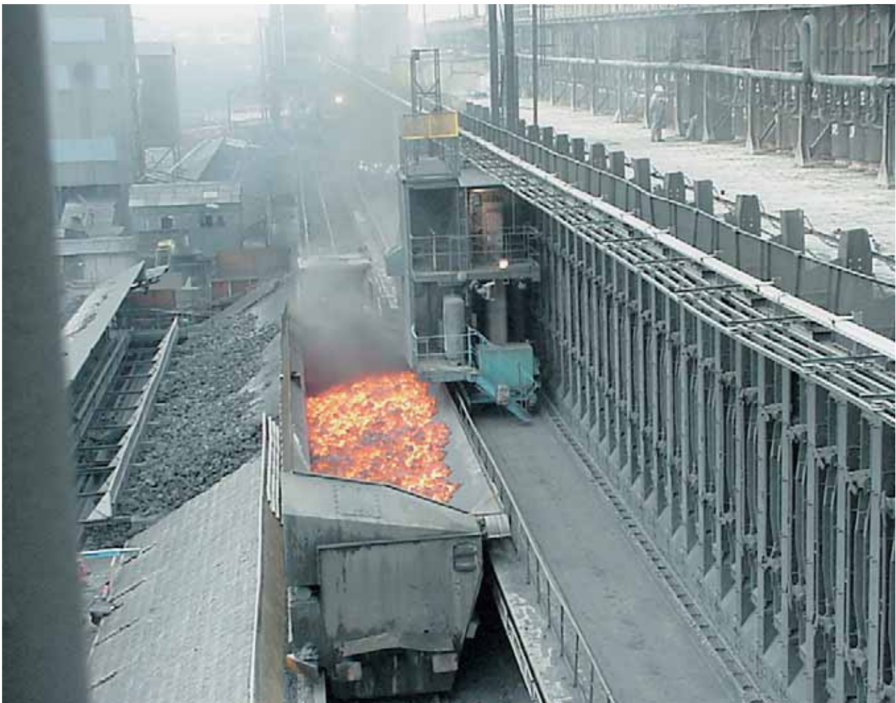
SMG in action for Ethernet data transmission for coking machinery
